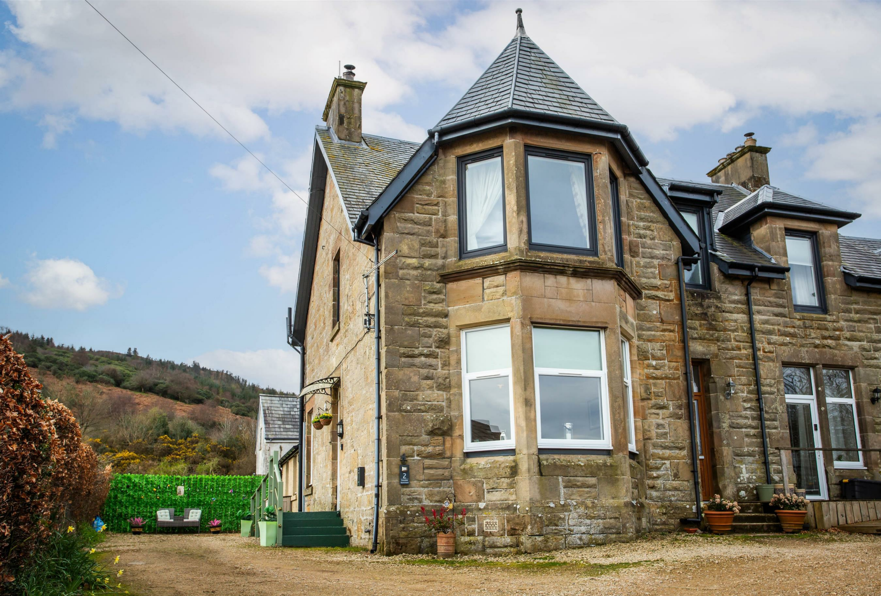
Apartment 2, Eaisdale House, Shore Road, Whiting Bay, KA27 8QW
